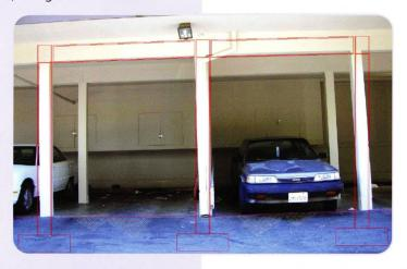
The use of a moment frame is indicated in red above to show how existing garages will be upgraded to improve their strength and better prevent damage in events such as earthquakes.
