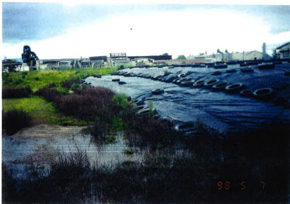
View of stockpiled contaminated soil, 1990 Bay Road site. (left)
