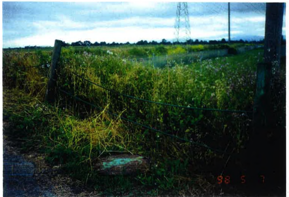
East Palo Alto Sanitary District (EPASD) manhole T23, located near northeastern corner of the subject Property. (right)
