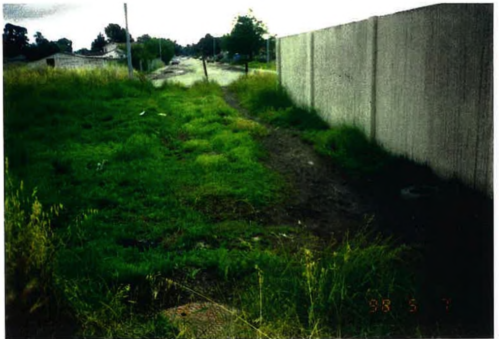
EPASD manhole T25 near eastern end of Weeks Street. (right)
