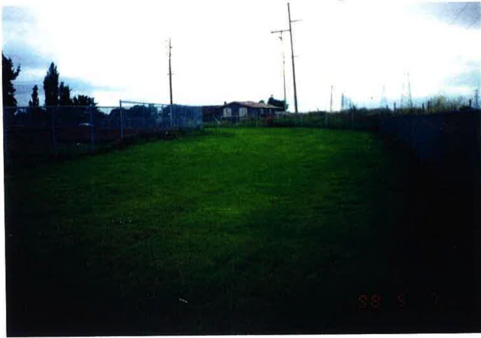
View of arsenic contamination cleanup area (foreground) from the east central portion of the subject Property. (left)
