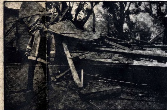
ALL THAT REMAINS — Thomas Smith, a Menlo Park firefighter, walks through rubble where tank stood.
