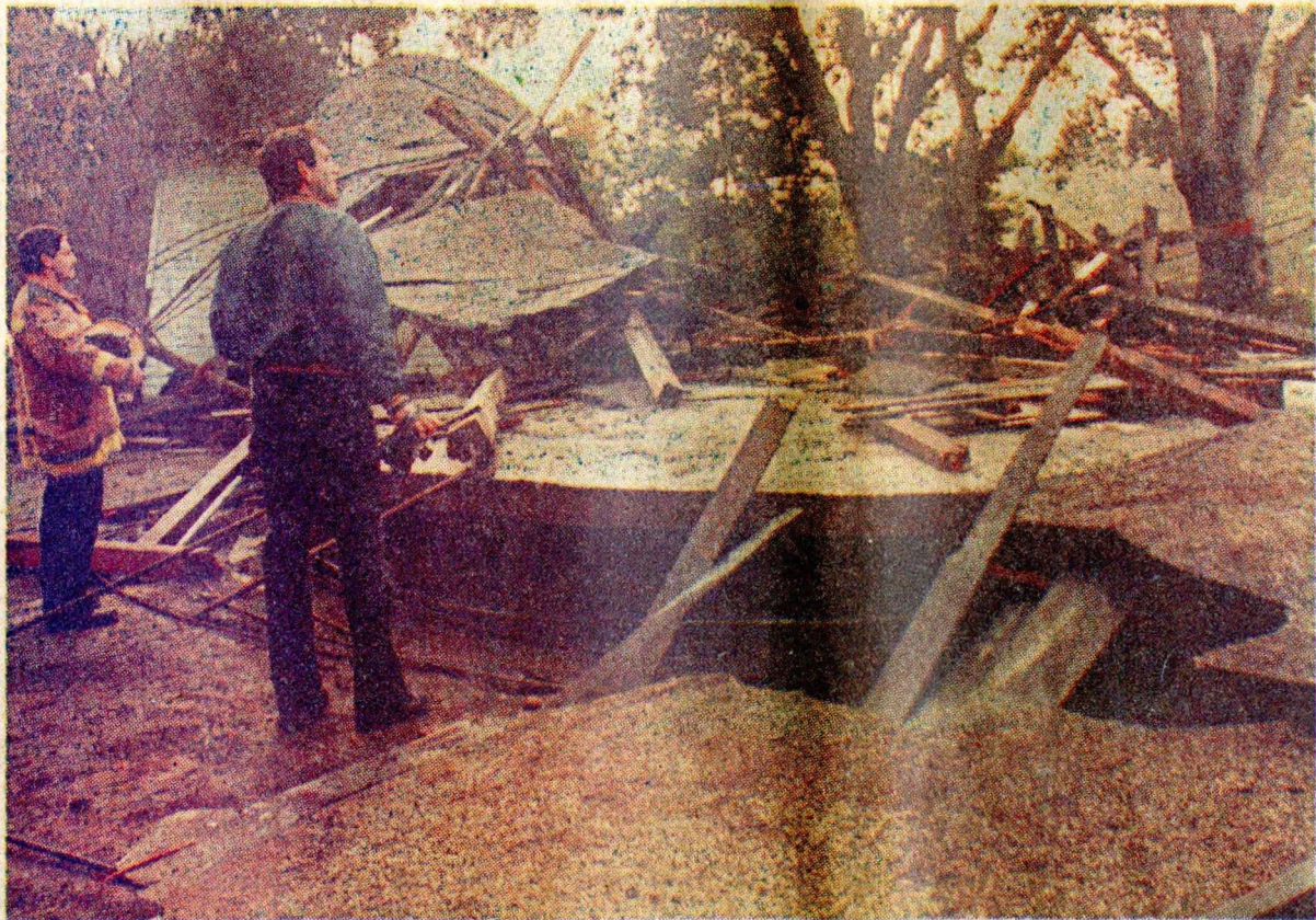
Menlo Park firefighter Ben Marra (left) and engineer George Miller survey a water tank that burst Wednesday afternoon in East Palo Alto, spilling 100,000 gallons. Details, B-1.
