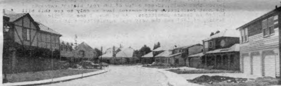
THE PALO ALTO UNIFIED SCHOOL DISTRICT SOLD VACANT LOTS AT THE SITE OF ABANDONED CRESCENT PARK ELEMENTARY SCHOOL FOR AN ESTIMATED FIVE MILLION DOLLARS. CONSTRUCTION OF THE TWENTY-EIGHT HOMES, TWO BLOCKS FROM EAST PALO ALTO, WILL ADD APPROXIMATELY FOURTEEN MILLION DOLLARS TO THE TAX ROLLS OF PALO ALTO. THIRD HOUSE ON RIGHT IS FOR LOW-INCOME.
